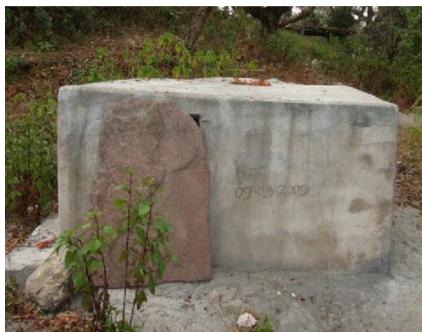
Figure 12: A cist renovated with cement and mortar
