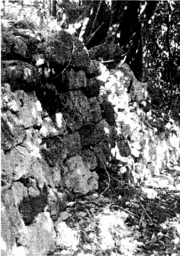
Figure 5: Keyed south wall, Chatan Gusuku. To NE.
