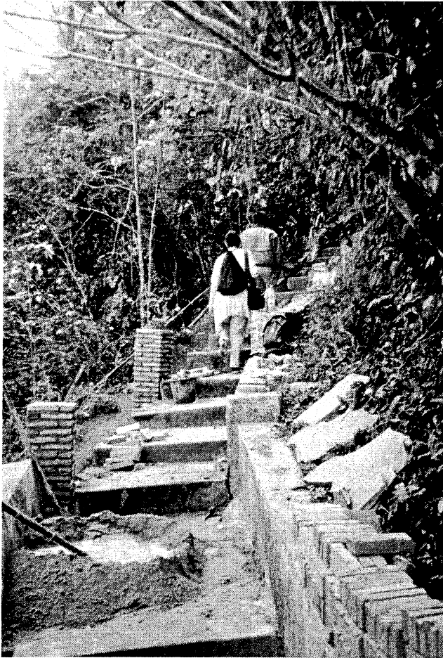
Figure 10: Walkway between the lower cave and the upper cave being reconstructed.
