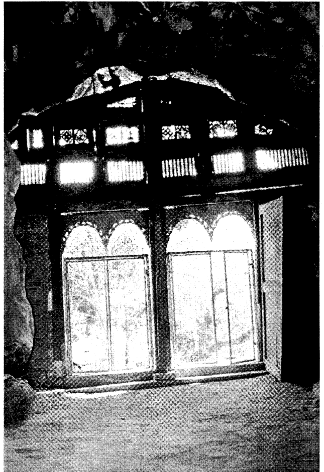
Figure 7: Entry to the upper cave, viewed from the interior, prior to being restored. The door to the left is laying to the side and the door to the right is cemented into the door step.
