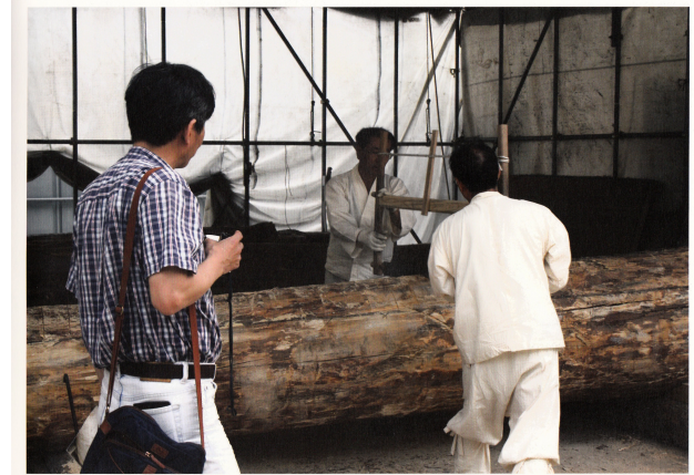
Figure 7. Carpenters in Korean dress using traditional tools to prepare domestic pine trees (Source: CHA 2011).
