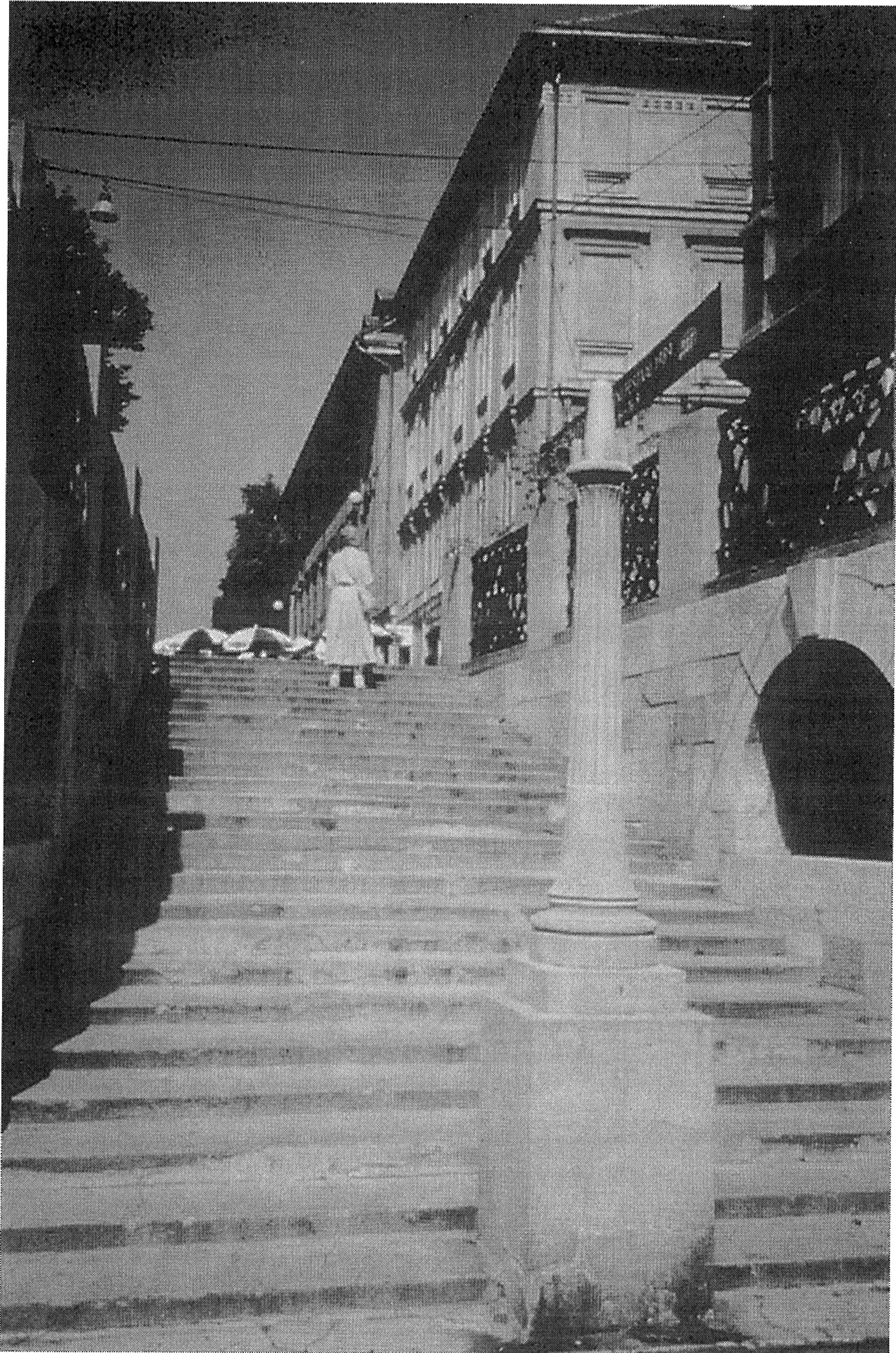
Fig. 5. The Gerber staircase from Congress Square to the Ljubljanica.
